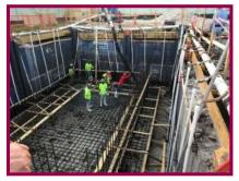
during construction. In addition to a heavier reinforcing design, we specify special underdrains, and a foundation pump to keep the water out of the "basement."
